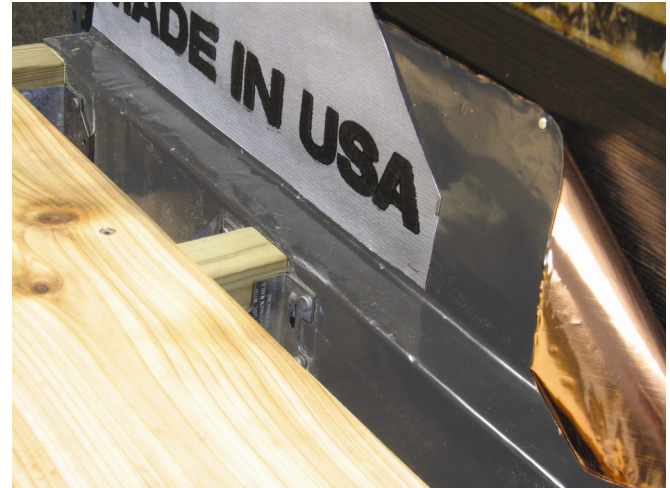
Cop-R-Shield PC should be installed with the copper side facing the plywood sheathing and the poly facing out.
