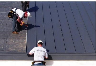
A hydrokinetic metal roof is sometimes used for commercial applications. It is attached to a corrugated metal roof deck with a layer of rigid insulation, typically between the metal deck and the metal roof.
