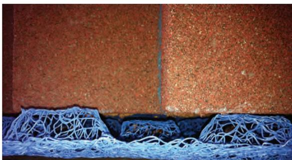
Overhead view shows the offset dimple design that breaks up mortar droppings on multiple levels.
